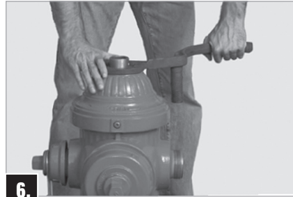
6. Remove Hold Down Nut, using Combination Spanner Wrench by turning counter-clockwise .
