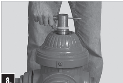
8. Remove Revolving Nut by turning in hydrant opening direction. It is not necessary to remove the Anti-Friction Bearing from the Revolving nut.
