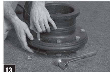
13. Place Flange Gasket onto top of Lower Standpipe and install Extension Standpipe using two Flange halves and eight Bolts and Nuts. Tighten (wrench tight) all bolts evenly.
