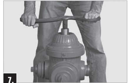
7. Use socket of Combination Wrench to remove Travel Stop Nut.
