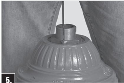
5. Using small Allen Wrench, loosen Hold Down Nut Set Screw.
