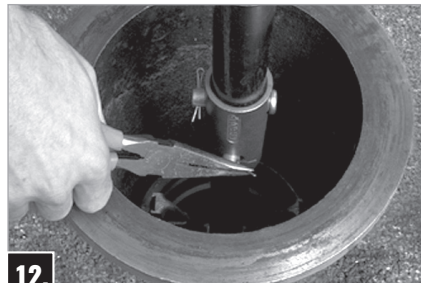
12. Install Rod Extension assembly onto the Lower Valve Rod and secure it with a Clevis Pin and Cotter Pin from the kit.
