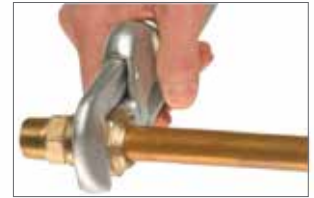
Insert the pipe and bottom out the nut.
