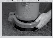
Assemble frangible Standpipe Coupling, making certain the bottom of the coupling is in its groove and that the top half of the coupling is uniformly engaged on the shoulder of the Upper Standpipe.
