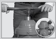
2 Using socket of Combination Spanner Wrench or %"thinwall socket, remove Travel Stop Nut. Remove Revolving Nut – turn in operating direction of hydrant. It is not necessary to separate the Anti-friction Bearing from Revolving Nut. Using a 7/32" Allen wrench, remove Bonnet Locking Screw. With the Combination Spanner Wrench, rotate Bonnet 22.5° (1/16 turn) counter-clockwise. As lugs disengage, lift the Bonnet off the Valve Rod.
