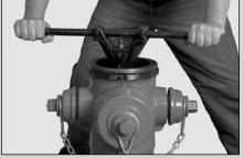
Reversing the above procedure, reinstall the Valve Rod and Main Valve assembly, fully threading it into the Seat Ring. To check for any leaks after being reinstalled, pull up on the Valve Rod to close the Main Valve—then, slowly open the auxiliary hydrant control valve to pressurize the elbow. Make sure seal is tight.
