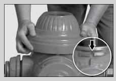
Replace the Bonnet Seal. Grease threads on Upper Valve Rod. Replace the Bonnet, turning clockwise into locked position. Next, grease the threads on Bonnet Locking Screw and reinstall. Be certain that the Bonnet is centered, so locking screw sets in the "V" of the locking slot in the Upper Standpipe.
