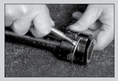
■ The hydrant can be restored to service without removing the bonnet or valve rod assembly by using the Traffic Repair Kit, which includes items 26-31, plus item 49, shown in drawing on Page 2. First, remove broken Valve Rod Coupling halves, Pins and Retaining Rings from Upper and Lower Valve Rod ends.
