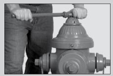
Slowly turn the Operating Nut in the closing direction, lowering the hydrant top section over the bottom section. Then, position the hydrant to face the proper direction. When the top section is aligned with the bottom section, continue to close until snug.
