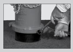
4 Retighten the Bolts and Nuts on the frangible Standpipe Coupling. Make sure to carefully tighten them to 50 ft-lbs torque, and the spaces between the ends of each coupling half are equal.
