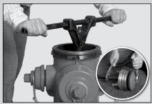
Remove Bonnet Seal. Using Seat Removal Wrench, unscrew the Valve Rod and Main Valve assembly, including bronze Seat Ring, by turning counterclockwise, and removing it as a unit. Holding Lower Valve Rod with a wrench, remove the Valve Bottom Plate.
