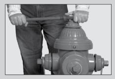
1 Open the hydrant Main Valve three turns.
