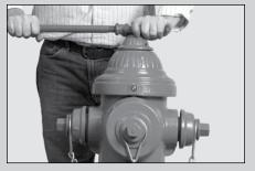
Make sure operating parts are clean and well lubricated before reassembly. Reassemble Bonnet onto extended Valve Rod assembly, following steps 7, 8 & 9 of the disassembly/reassembly procedure on Page 7.
