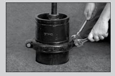
5 Install Extension Standpipe Coupling with stainless steel Bolts & Nuts, so the grooves in both the Lower Standpipe and Extension are engaged equally, and bolts are tightened to 50 ft-lbs torque, and the space between ends of coupling are equal on both sides of hydrant.
