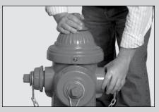
Check pressure tightness of reassembled parts by following steps 2, 3 & 4 of AWWA certified inspection procedure. Following that, open the hydrant, allowing water to flow again. Close and check for proper drainage. If no problems are evident, the hydrant is already closed and considered back in service.
