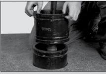
4 Clean grooves in Lower Standpipe and Extension section. Install the Extension Coupling Gasket in groove on the bottom of the Extension. Either grease or gasket cement may be applied to keep it in place. Position the Extension over the Lower Standpipe.
