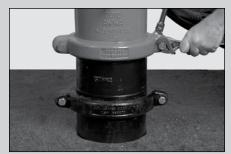
Reassemble frangible Standpipe Coupling around lip of Upper Standpipe and groove in the Extension. Make certain that there is uniform engagement all around – then, carefully tighten the Coupling Bolts & Nuts to 50 ft-lbs torque, and the space on each side is equal.
