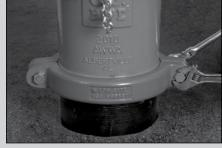
Carefully tighten the Coupling Bolts & Nuts to 50 ft-lbs torque, and the space on each side is equal. Operate hydrant and check for leaks.
