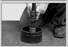
Install Rod Extension between Upper and Lower Valve Rods, making sure that the non-frangible Extension Rod Coupling (without break groove) is below, and the frangible Valve Rod Coupling (with groove) is above. Be sure to reinstall Dampener ring between Extension and Frangible Couplings. Replace all Pins and secure each with stainless steel Coupling Retainer Rings.
